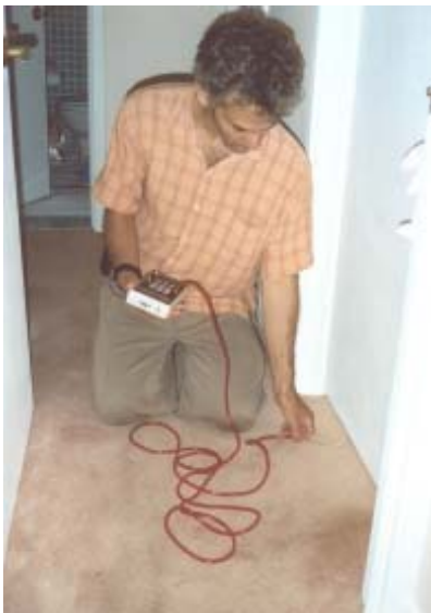
Walder uses a pressure meter to measure the air pressure in a bedroom as part of a combustion gas safety test.
