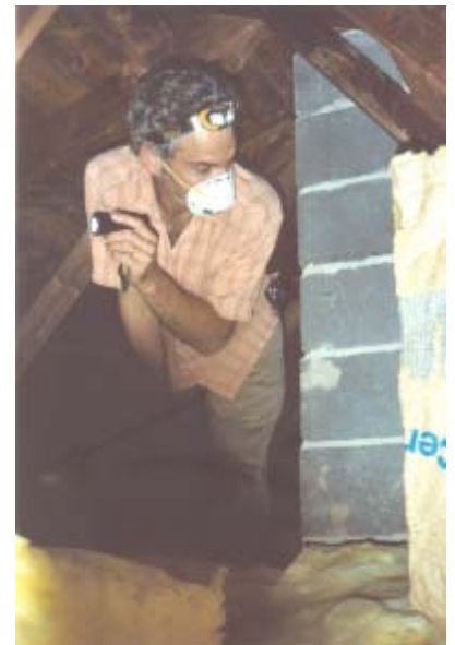
Walder checks the attic.
