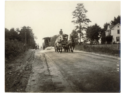
Road crews paving Rockville Pike with macadam in the late 19th century.
