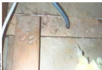
*A home energy audit can reveal problems such as a shrunken top plate (shown above) in an attic. These wooden boards are installed horizontally above the studs to support the rafters. When they shrink over time, they let interior heated air escape into the attic in winter.*
